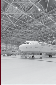
Turkish Airlines Additional Facility for Istanbul Airport, Turkey
